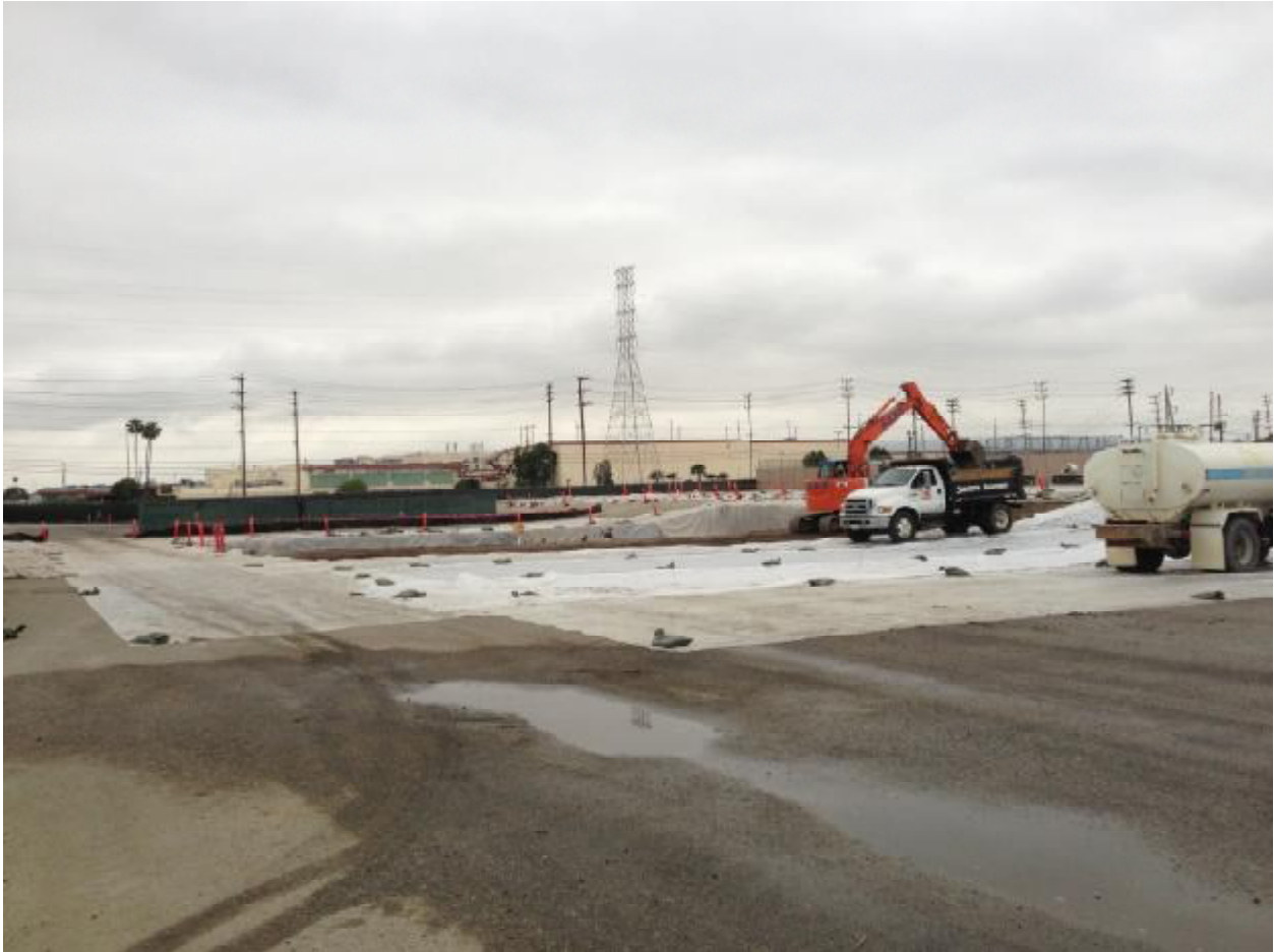
Excavation area. Taken facing southwest.
