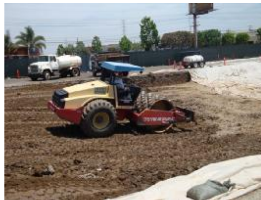
Compacting Soil under treatment pad area (5/21/2013)
