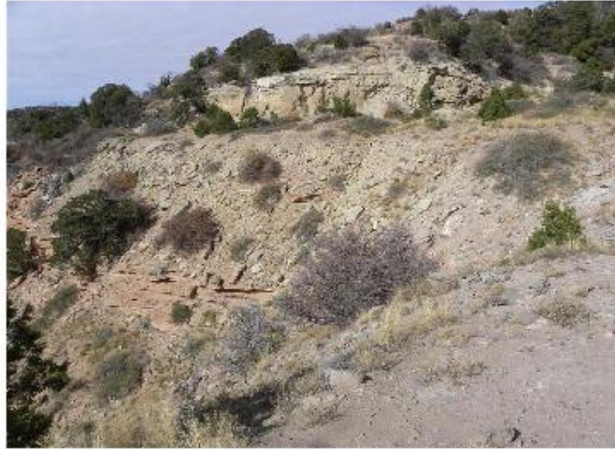
Photo 7. Waste debris sloughing down slope
