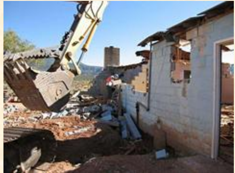
Contaminated Structure Removal
