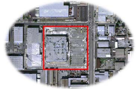
An aerial view of the former Discount Priceland site in Gardena, California.
