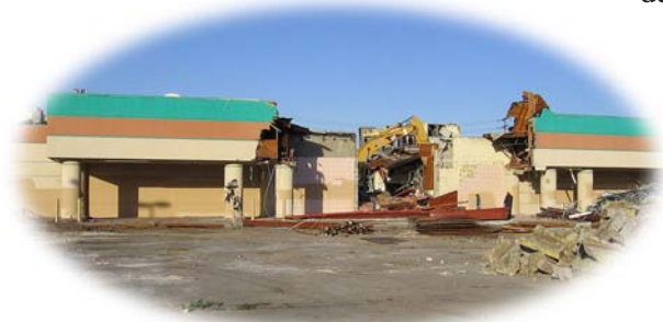
Demolition in progress on the former Discount Priceland site.
