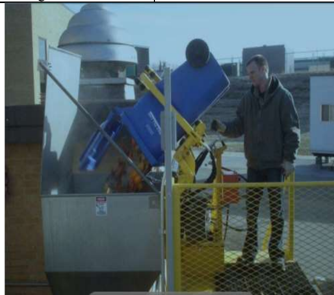
At the West Lafayette WRRF, an operator stands by as the cart tipper empties a toter into the hopper.
