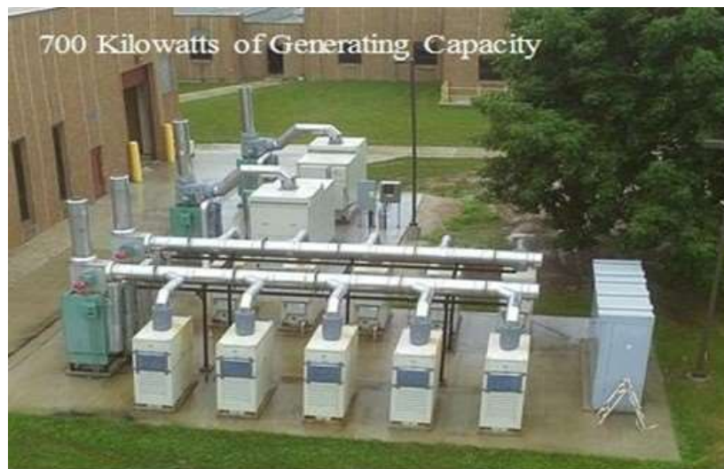
Figure 9: Microturbines at the Sheboygan WRRF Source: Sheboygan Regional Wastewater Treatment Facility 2011
