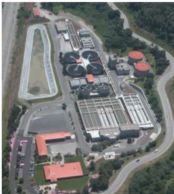
Photo provided courtesy of CMSA
