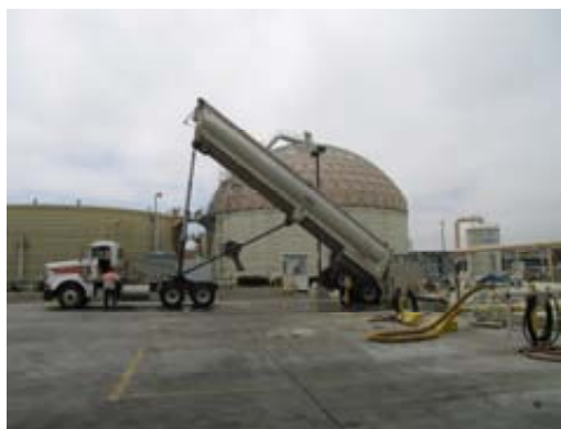
Food waste is delivered to EBMUD and screened, ground and cleaned of contaminants. A typical delivery is approximately 20 tons total weight.
