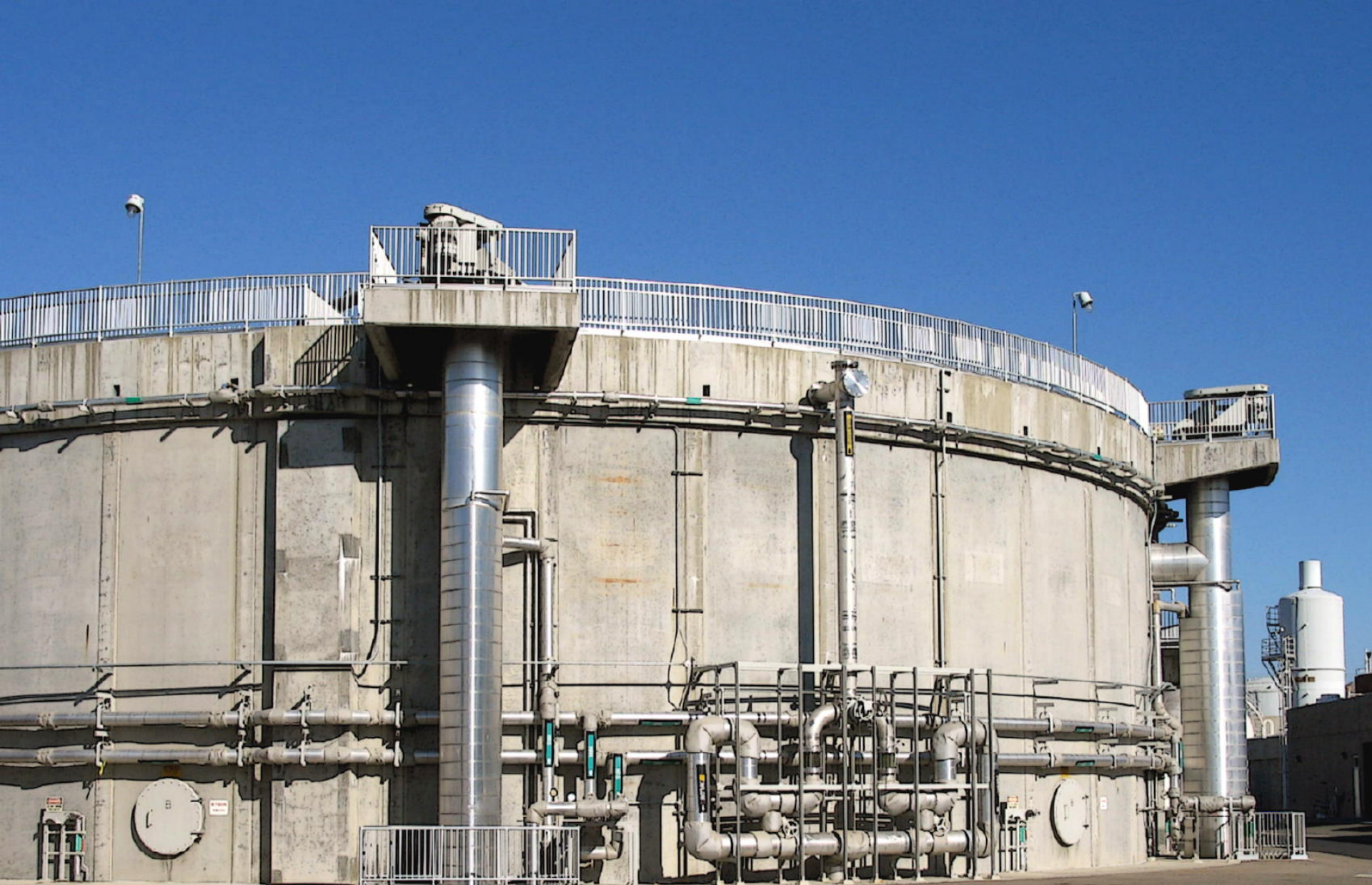
Anaerobic Digester with external Draft Tube mixers Constructed in 1996
