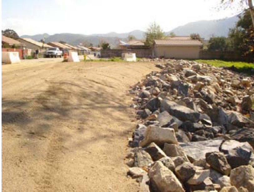
Figure 4 View of bermed embankment along Pala Creek, south of Nejo Road (2/26/09)
