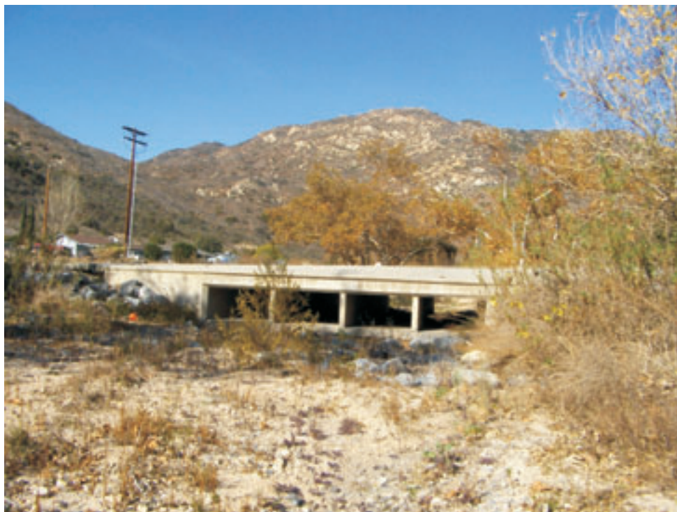
View of Sycamore Lane crossing of Pala Creek, looking north (12/22/05)
