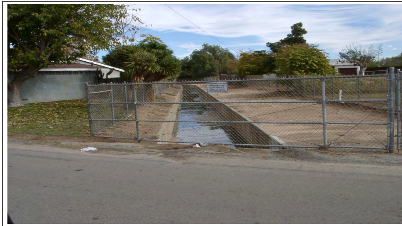
View to northeast of concrete drainage channel along Edgemont Street
