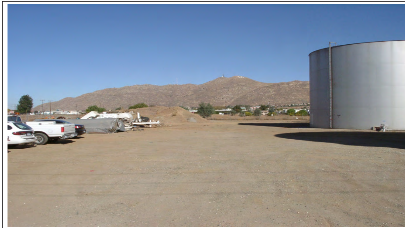
View to north from tank, booster, well site
