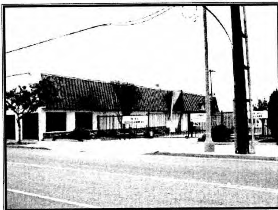
Figure 18. Building west of 14 th Street.
