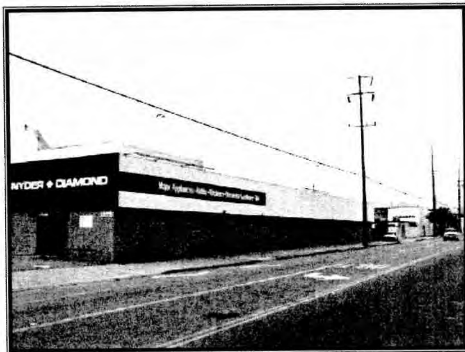
Figure 17. Building north of intersection of 14 th Street and Olympic Boulevard.
