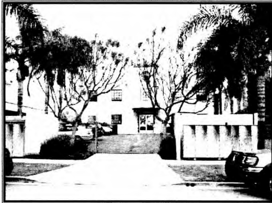
Figure 12. Building southeast of the intersection of Colorado Boulevard and 16 th Street.
