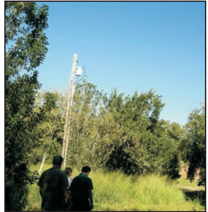
Existing overhead electrical line on the property.
