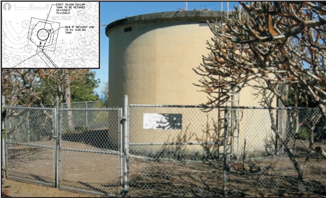
Existing DWS 0.05 MG Kapulena Homestead Reservoir.
