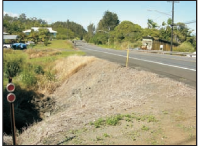
B. Honoka'a-Waipio Road from entry looking north.
