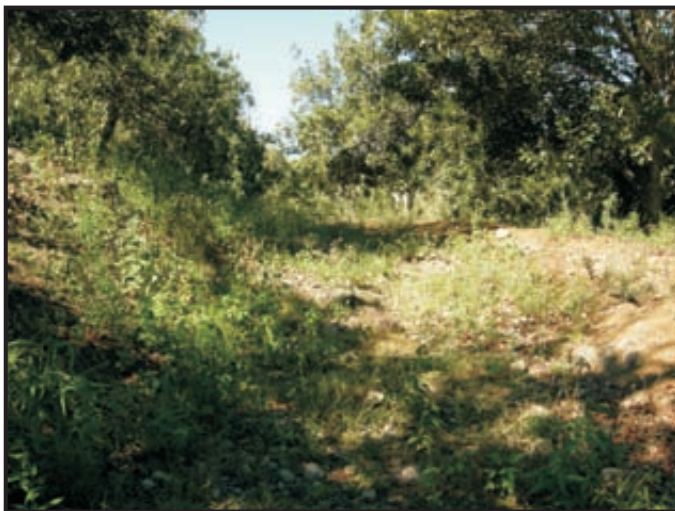
C. Existing driveway to be upgraded to access to the project site..
