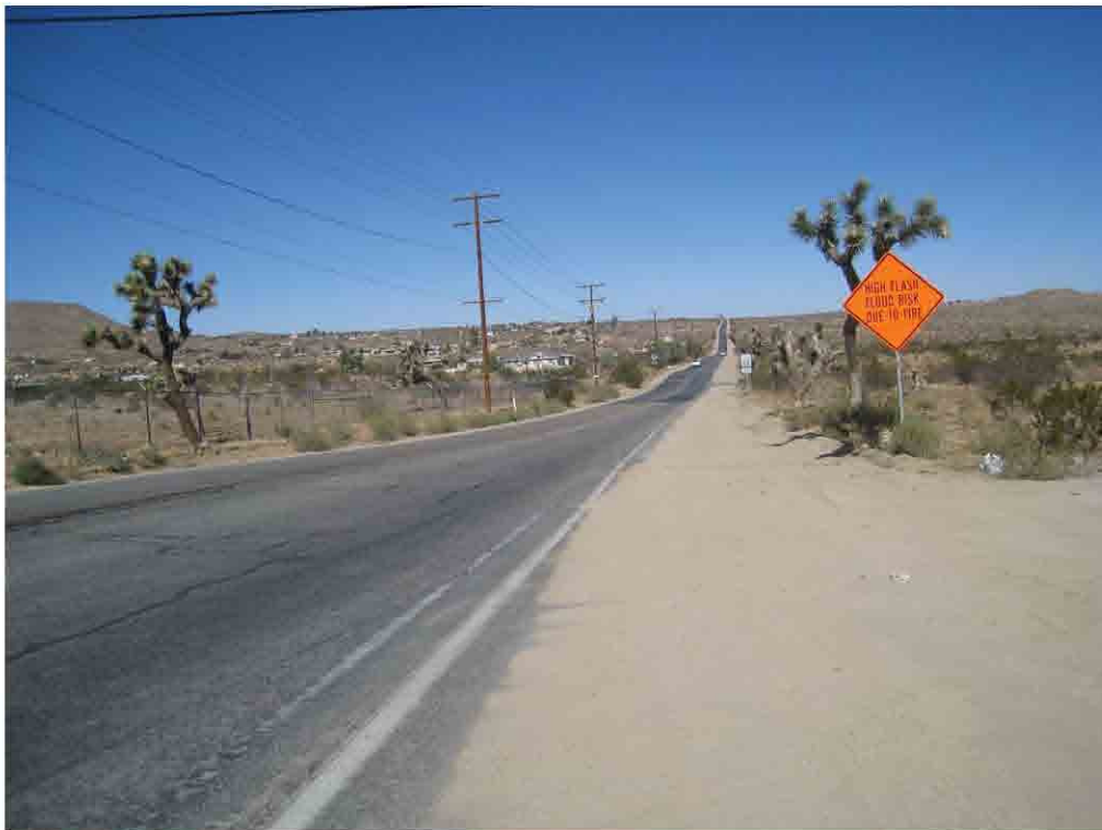
Pipeline Route – View looking north along Yucca Mesa Road from State Route 62
