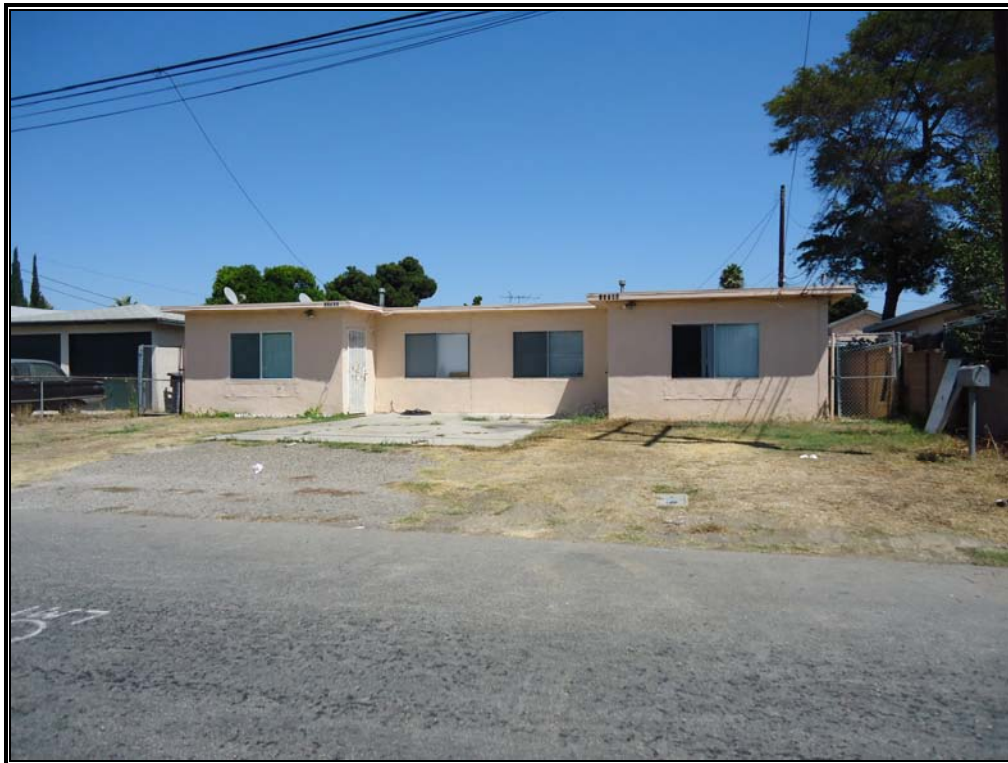
Figure 8 Example of no curb or gutter. Northern end of Pacific Avenue near 21 st Street.
