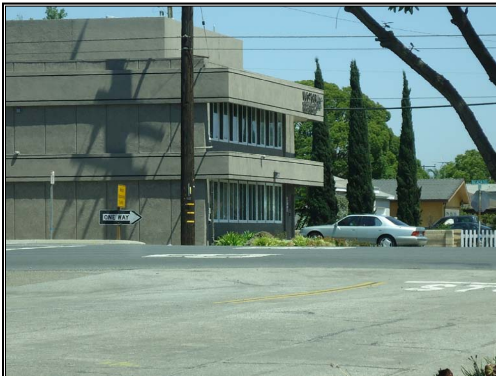
Figure 10 View east toward Beach Blvd. from 19 th Street. Note super-elevation of Beach Blvd.
