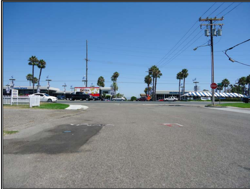
Figure 9 View east toward Beach Blvd. from 23 rd Street. Note super-elevation of Beach Blvd.
