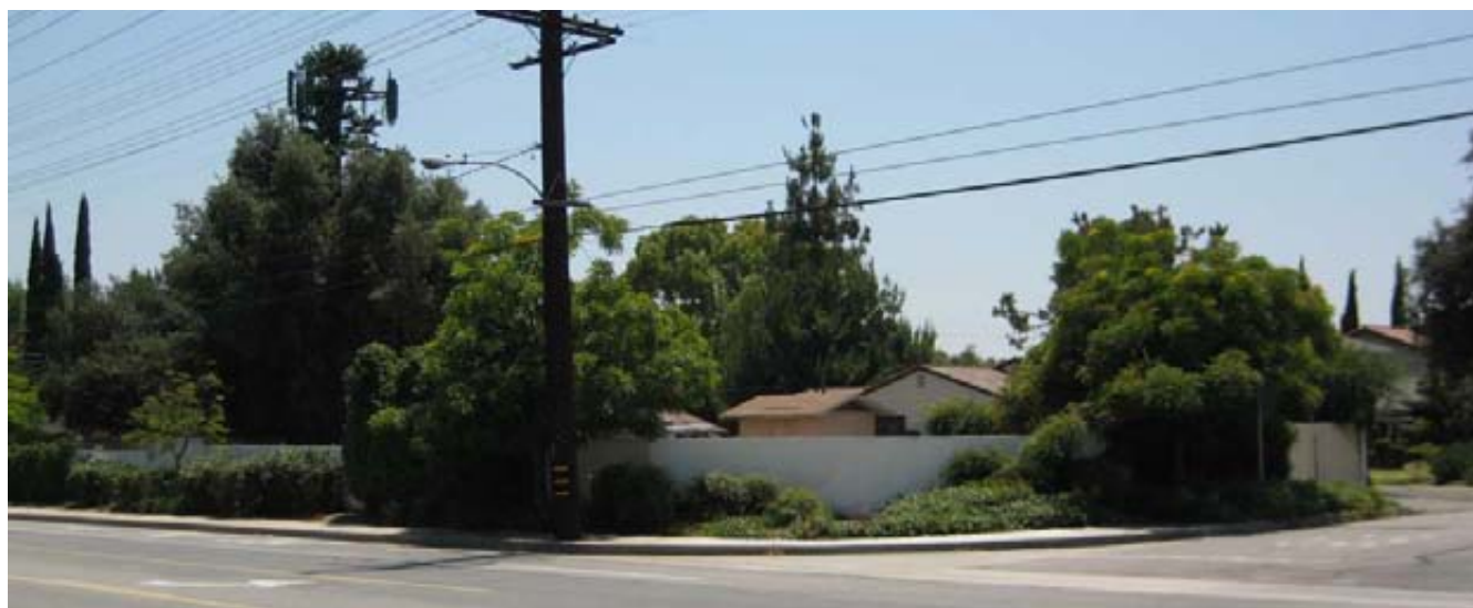
FIGURE 6 VIEW OF LONGLEY FACILITY LOOKING SOUTHWEST FROM EL MONTE AVENUE
