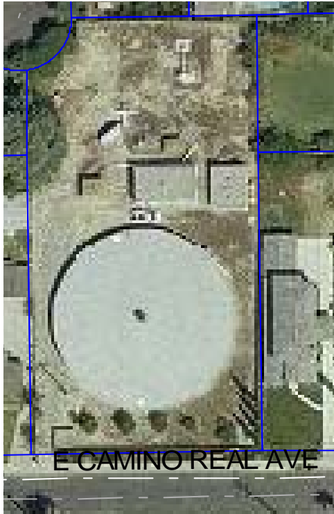
FIGURE 8 AERIAL VIEW OF CAMINO REAL
