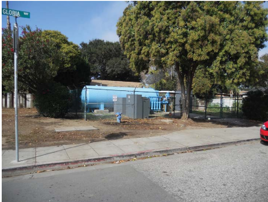
Figure 2: Gloria Way Well Site
