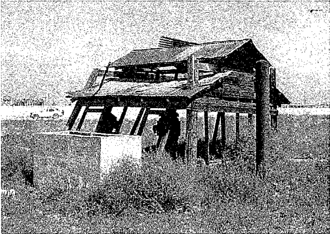
Photograph 25. City of Redlands Well #2.
