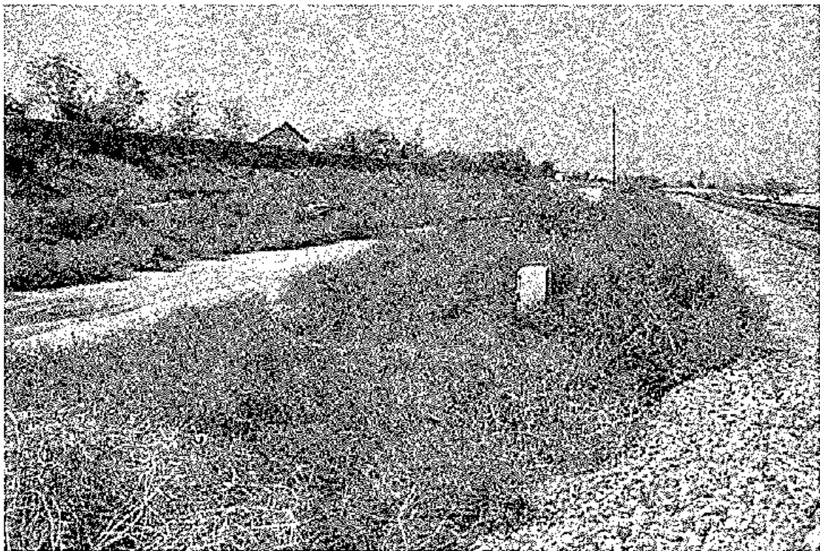
Photograph 20. View of properties adjacent to the railroad tracks and the creek.
