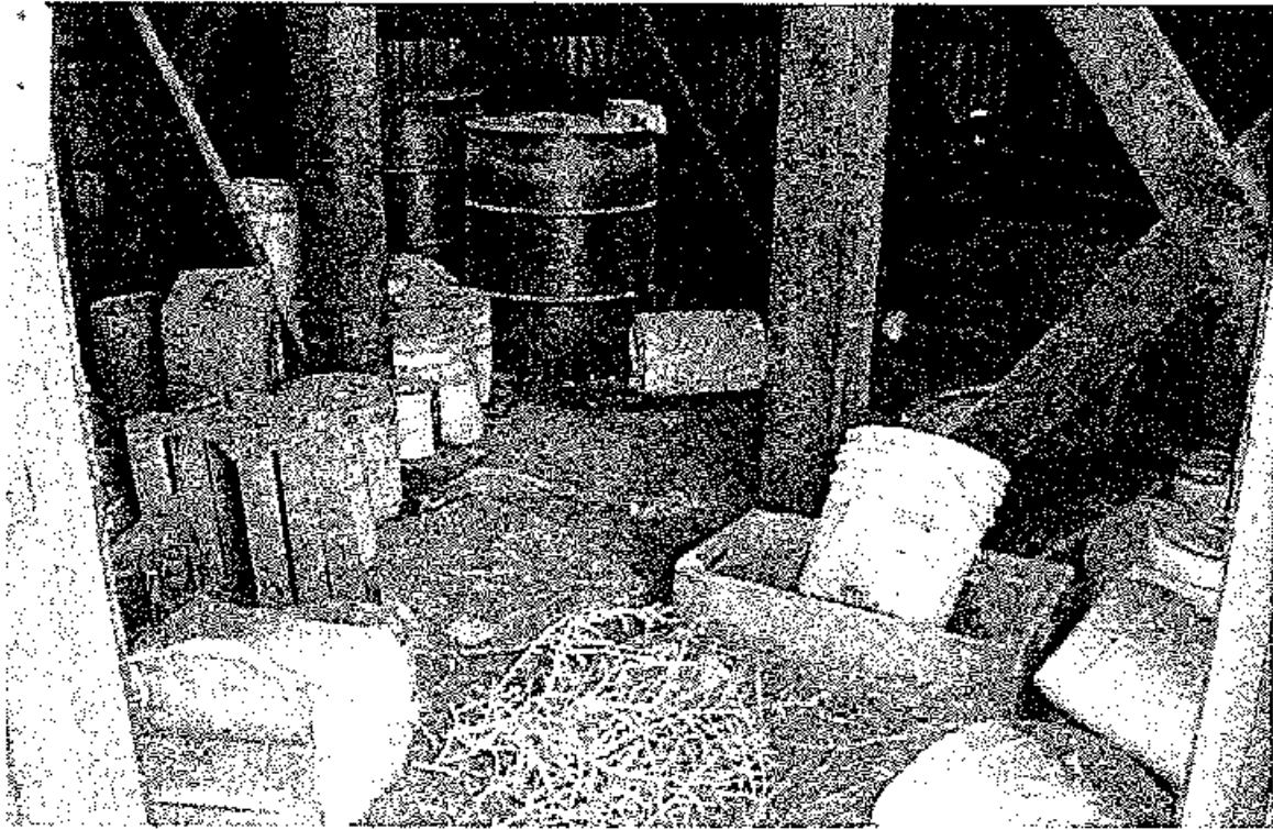
Photograph 35. Looking inside the water tank adjacent to three aboveground oil tanks.
