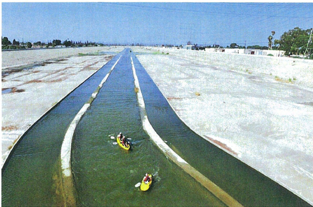
Figure 3. Photographs from July 25-27, 2008, taken by members of the Los Angeles River Expedition during the mid-point of the dry season. Examples of low flow channels embedded with larger concrete-lined flood channel. Top: Near the confluence of Arroyo Seco at the Interstate 110 overcrossing (RM 24.7). Bottom: Typical 16-mile reach between Vernon and Long Beach (RM 3.2-19.2).
