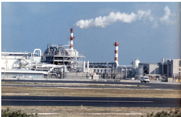
JACADS facility with incinerators inside
