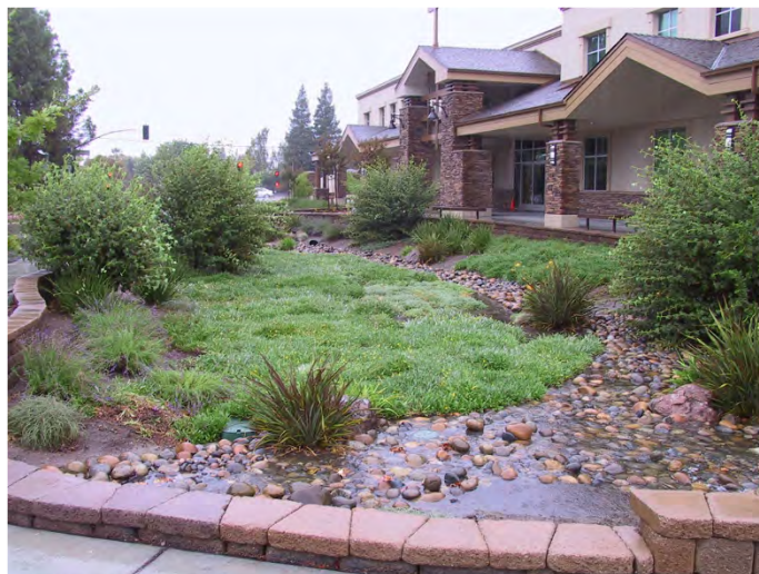
Bioretention facility treats runoff. Photo by Scott Wikstrom, City of Walnut Creek
