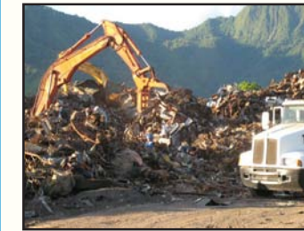
Cleanup crews remove scrap metal from yard
