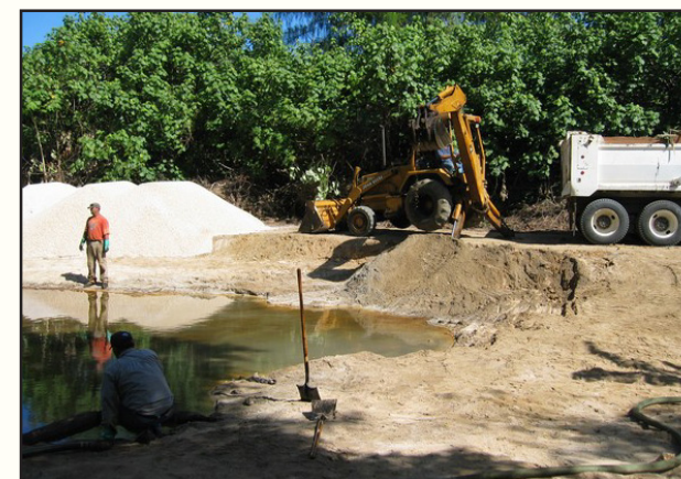
Contaminated soil removal from site
