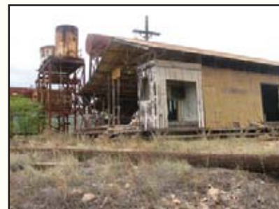
Debris from former activity on site
