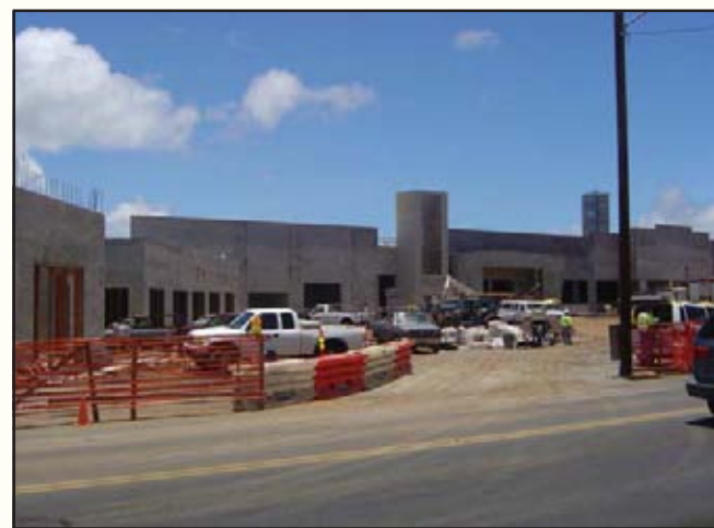
Redevelopment construction for new Safeway and retail complex
