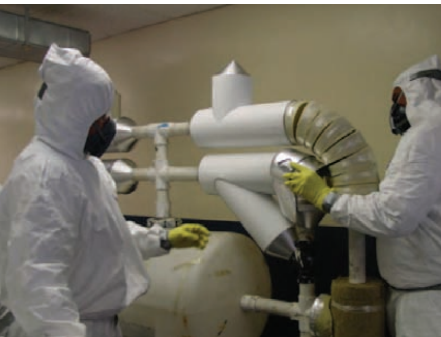
Left: Trainees learning asbestos abatement techniques.
