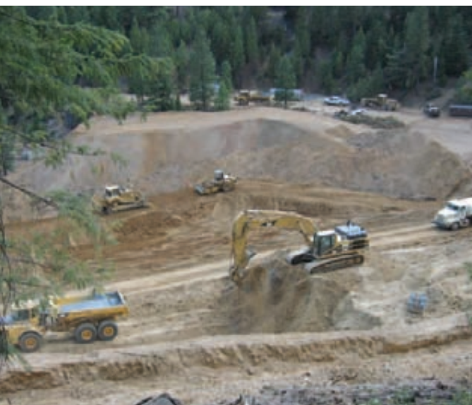
Left: Heavy equipment prepares disposal site for mercury-contaminated mining waste removed from creekbed.
