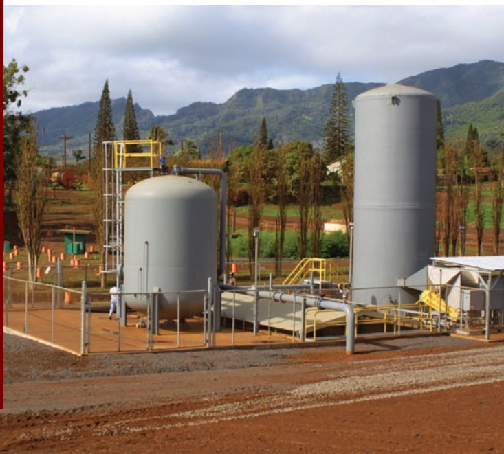
Groundwater treatment system at the Del Monte Superfund site, Kunia, Hawaii.
