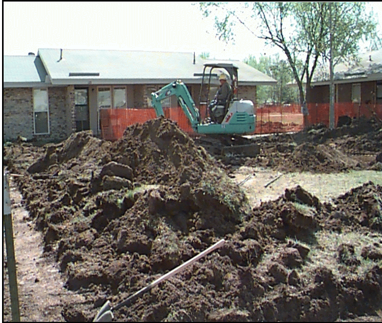
Excavation of Contaminated Soils From A Residential Area
