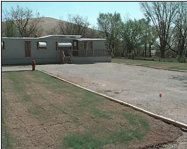
Remediated Property - Note the chat pile in the background and the recently placed sod and limestone driveway in the foreground.
