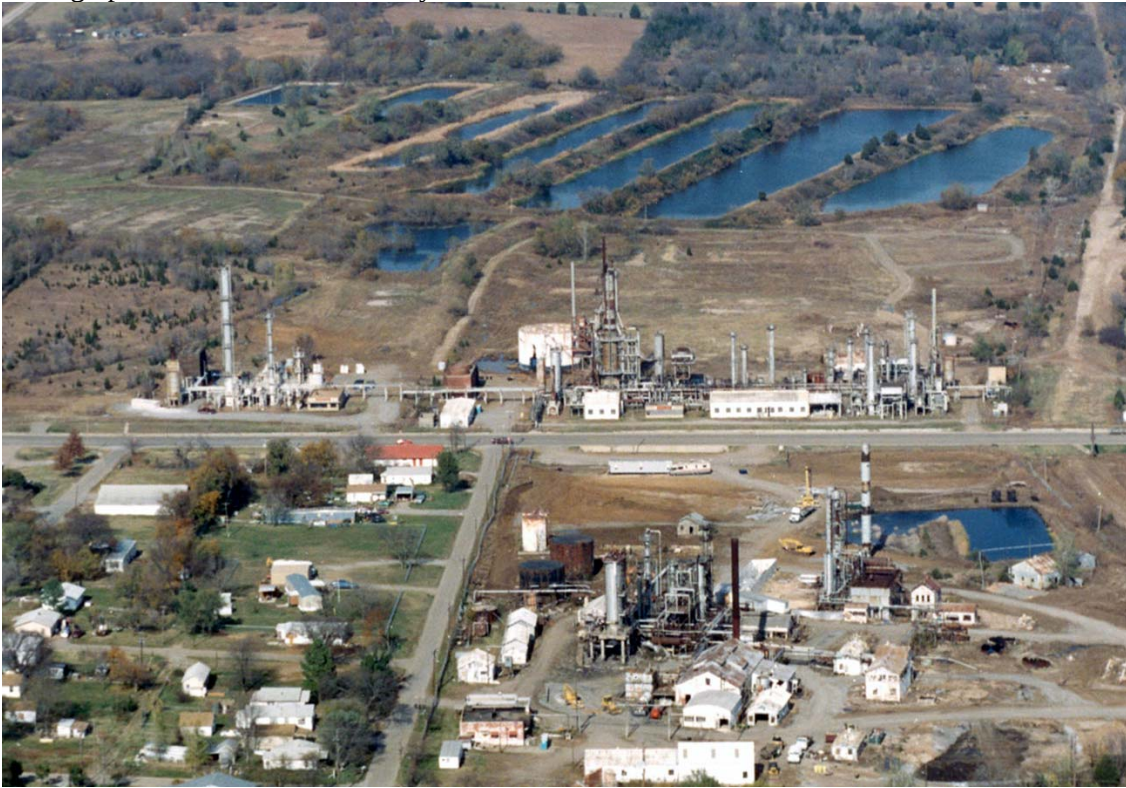
Photograph 2 – Abandoned Refinery Prior to Removal Actions
