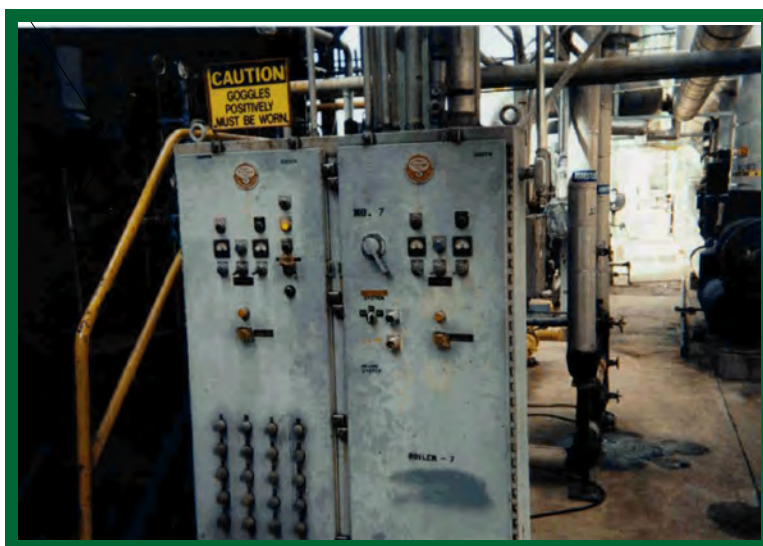
Local control panels often include meters and local data readouts that should also have calibration records.
