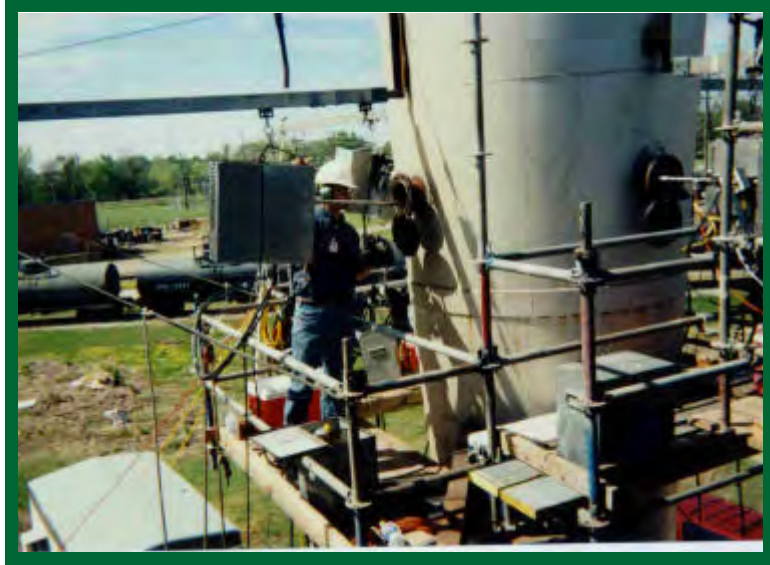
This photograph shows a Method 0050 sampling train being pushed into the sample port. The observer should check to ensure that the probe is properly positioned at each sampling location.
