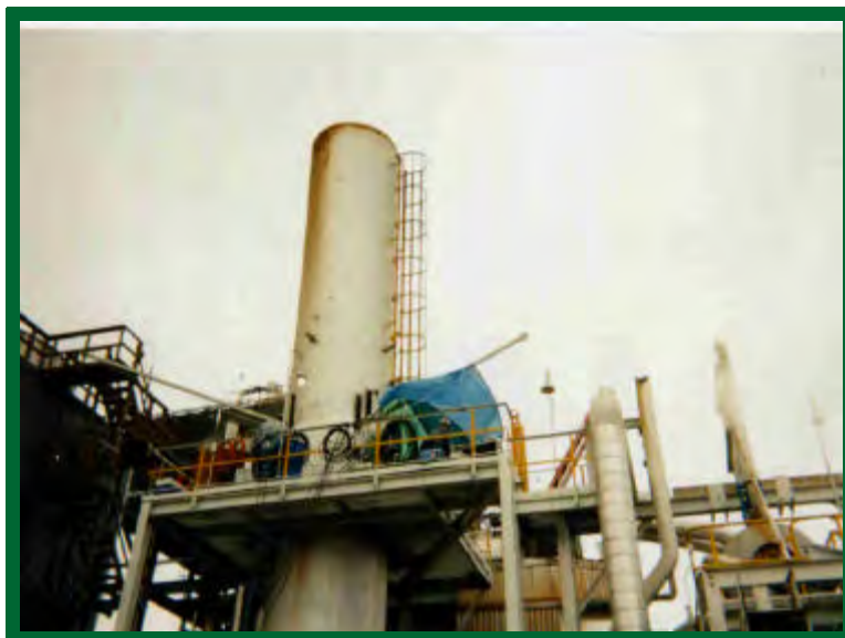
This stack measures 4.7 square meters (50 square feet in cross-sectional area and 18 meters [60 feet] high). The oversight team should verify the dimensions of each stack.
