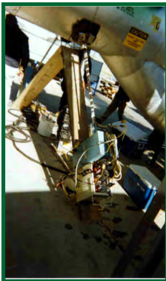
Stack sampling ports on this horizontal duct are placed at a 90 degree angle to each other.
