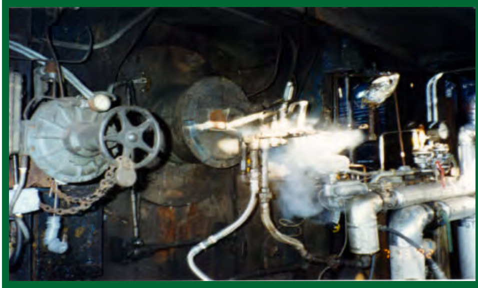
Example feed end of a combustion unit, showing waste feed guns
