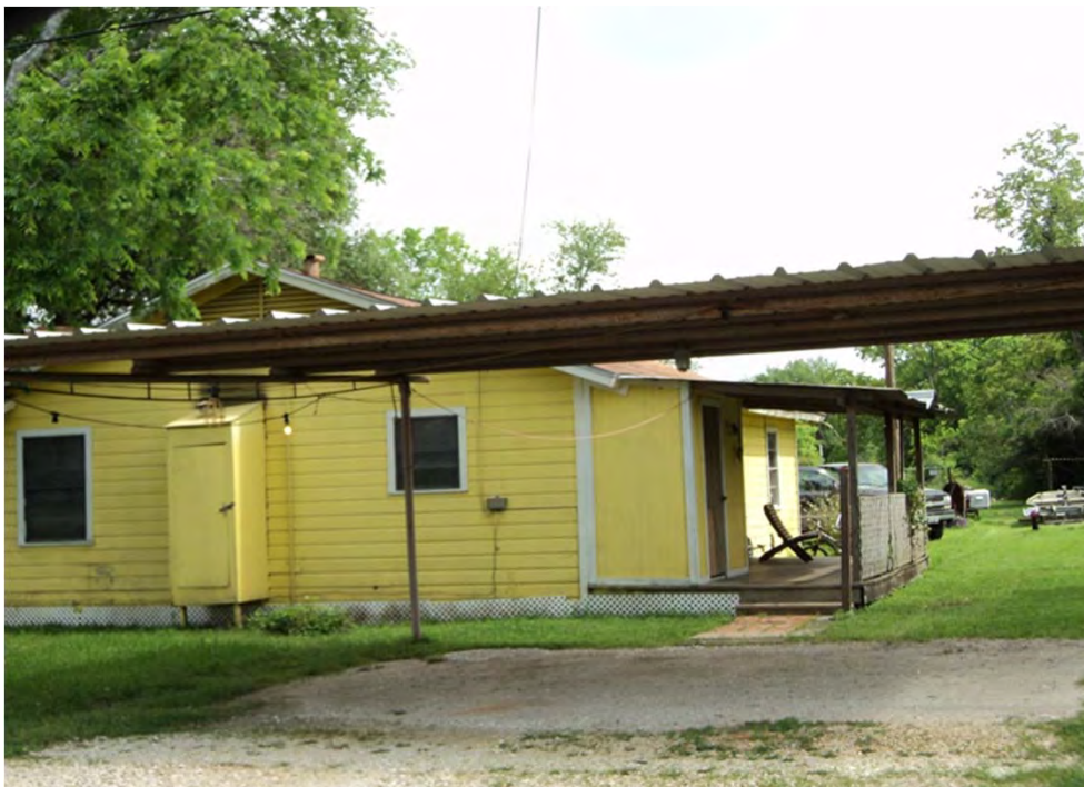
Photograph 9: Structure 2 along Winfree Avenue, facing south.
