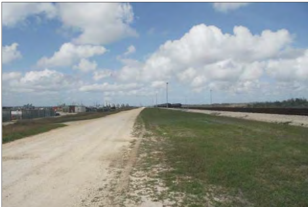
Plate A4. General overview of development within the southeastern portion of the Consultation Area/APE north of FM 4321. Photograph taken in February of 2012. View is to the north.
