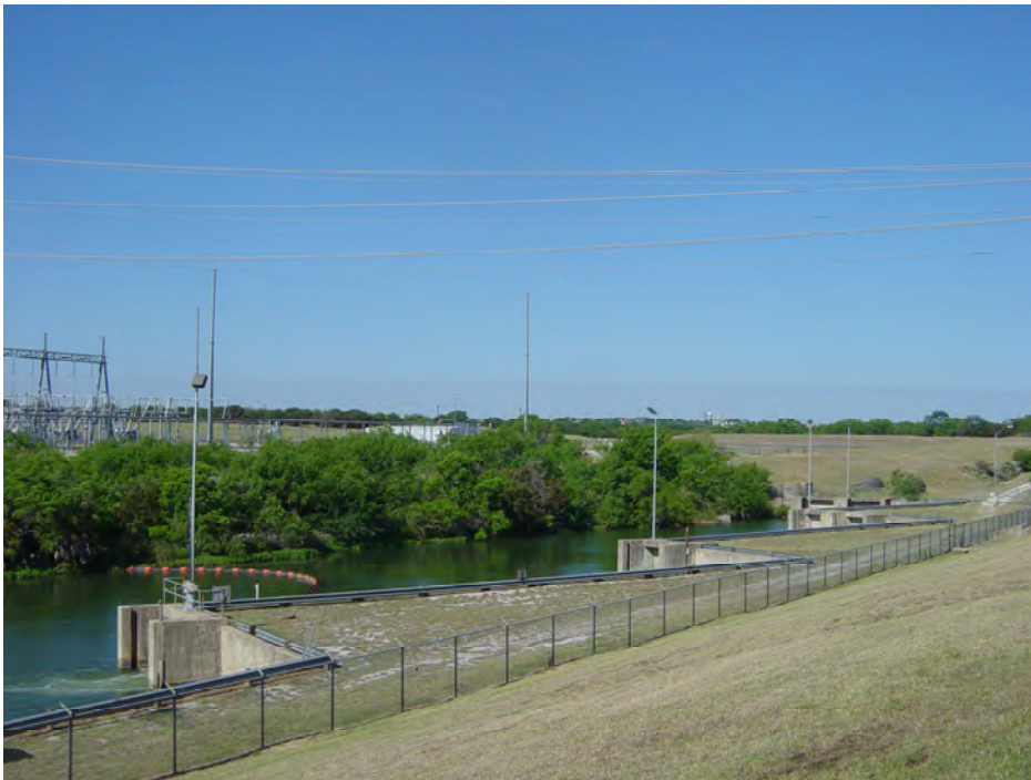
Photo 2 Wastewater Discharge Facility
