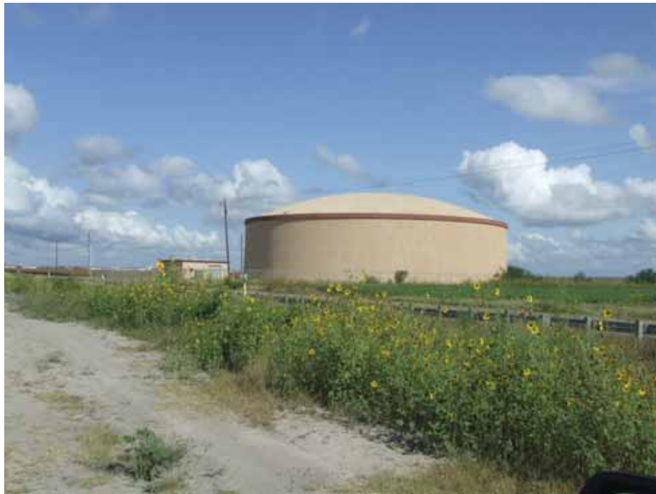
Photograph 10: June 7, 2012 View of established infrastructure to NW of proposed construction site.
