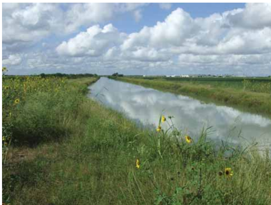
Photograph 6: June 7, 2012 Looking south from SW corner of proposed construction site.
