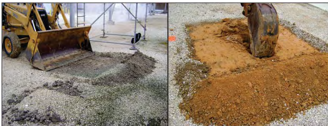
Figure 7. Removal of white gravel layer prior to test pit excavation. Note the difference in top soil (foundation) color. Moving across the AOE (approx. south-north) the soil color becomes lighter.
