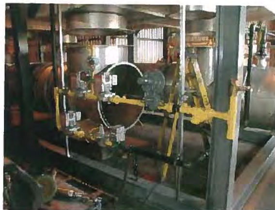
Supplemental Fuel Injection (SFI) Additional Fuel Train Piping
