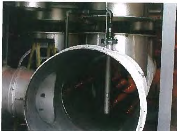
Supplemental Fuel Injection (SFI) Custom Designed Injection Quill
