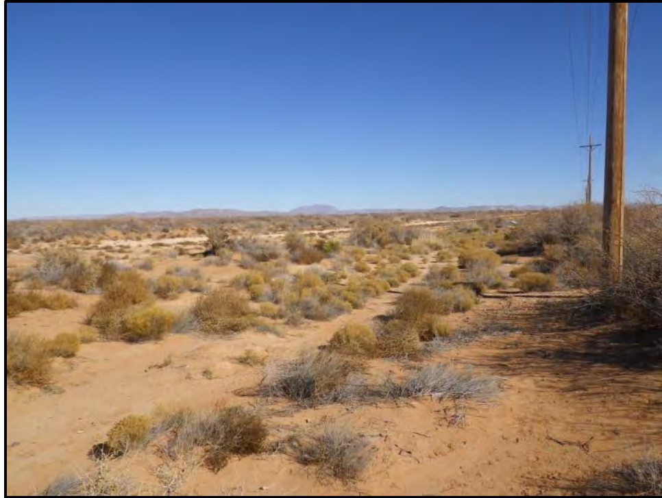
Photo C-1. DP1 – Typical vegetation near the Caliente Substation in the northwest portion of the project area; view facing east along Filing 2 of the proposed transmission line alternatives.
