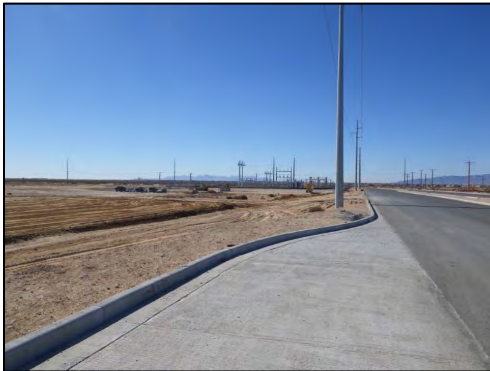
Photo C-23. PP9 – Taken in the southwestern end of the project area along the proposed transmission line alternative for Filing 3; view facing west towards the Montwood Substation.
