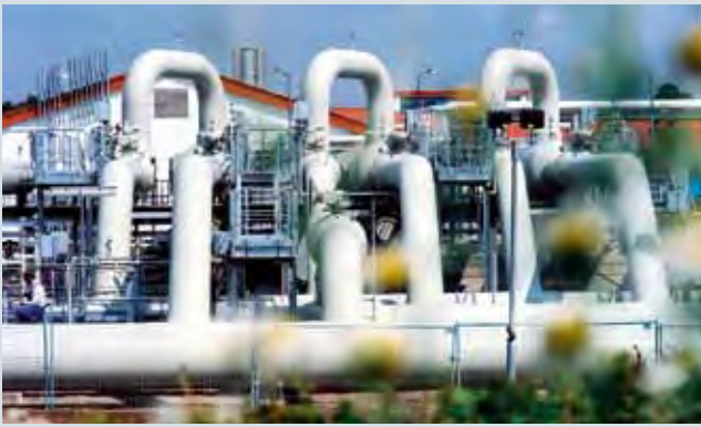
Wingas compressor station, Eischleben, Germany: Two Siemens compressor trains, each powered by a 30MW SGT-700 gas turbine, boosting the pipeline pressure for Natural gas* transport.
