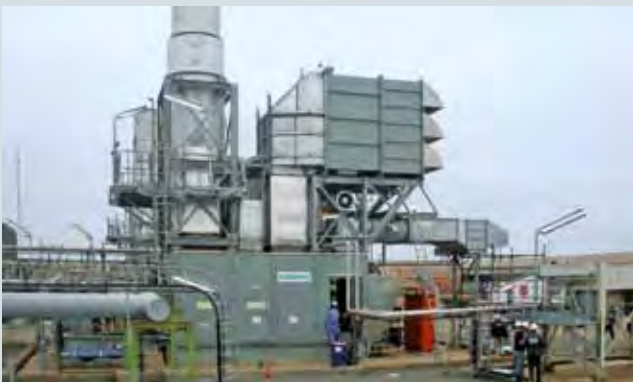
Sasol Technology (Pty) Ltd, South Africa: The 13.4MW SGT-400 gas turbine is the key component to the two pipeline compressor sets installed at the Komatipoort compressor station.
