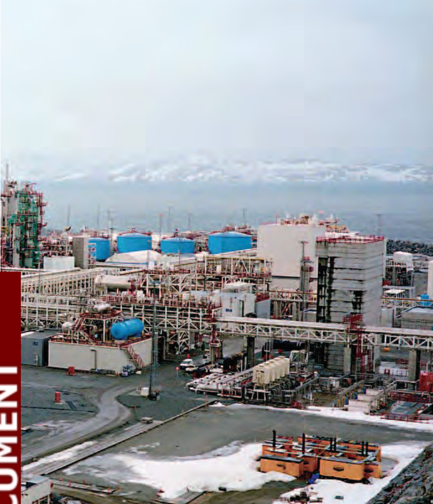
Statoil's Melkøya Island LNG plant near Hammerfest, Norway. The world's first all-electric LNG plant, its main refrigerant compressors are powered by two massive Siemens 65-megawatt variable-speed drive systems (VSDS). Siemens also delivered the compression solutions for methane mix and CO 2 re-injection.
