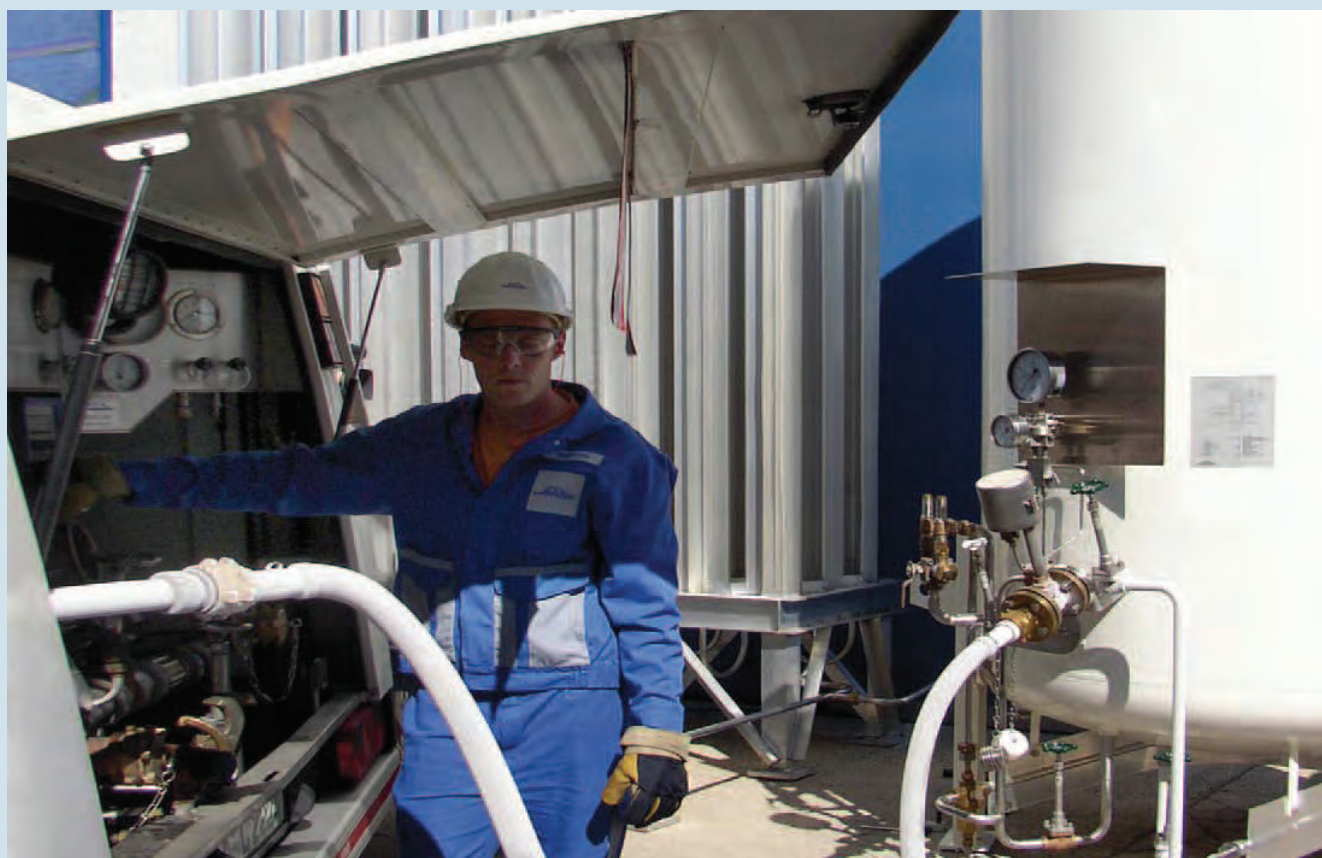
Truck unloading at LNG satellite station
