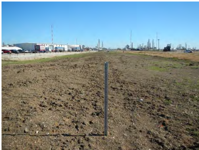
Photo 43- Western portion of the proposed pipeline rights-of-way south corridor with recent disturbance and no vegetation.
