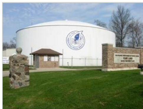
Storage, Flint Lake Drinking Water Plant
