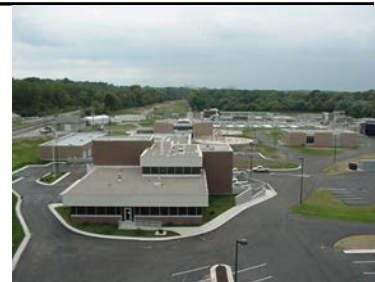
Lafayette Wastewater Treatment Plant
