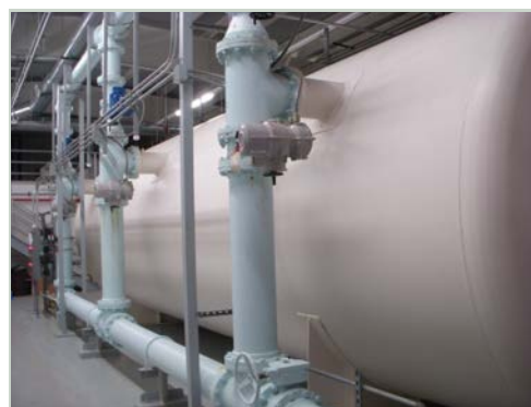
High Pressure Filtration, Flint Lake Drinking Water Plant
