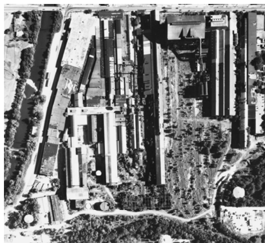
Pre-demolition photo, Main Plant Area, 1998
