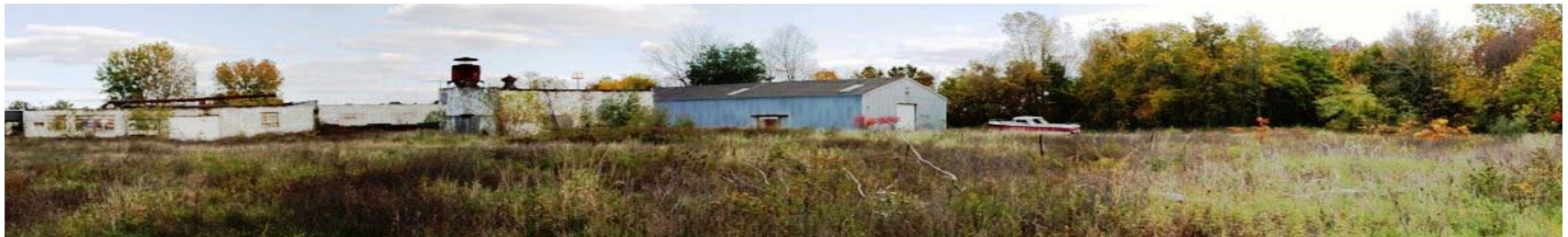
Abandoned Industrial Buildings in Paw Paw, Michigan
