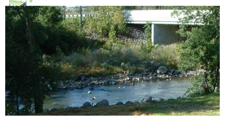
Large granite field stones removed from the topsoil layer, set aside, used to stabilize creek banks
