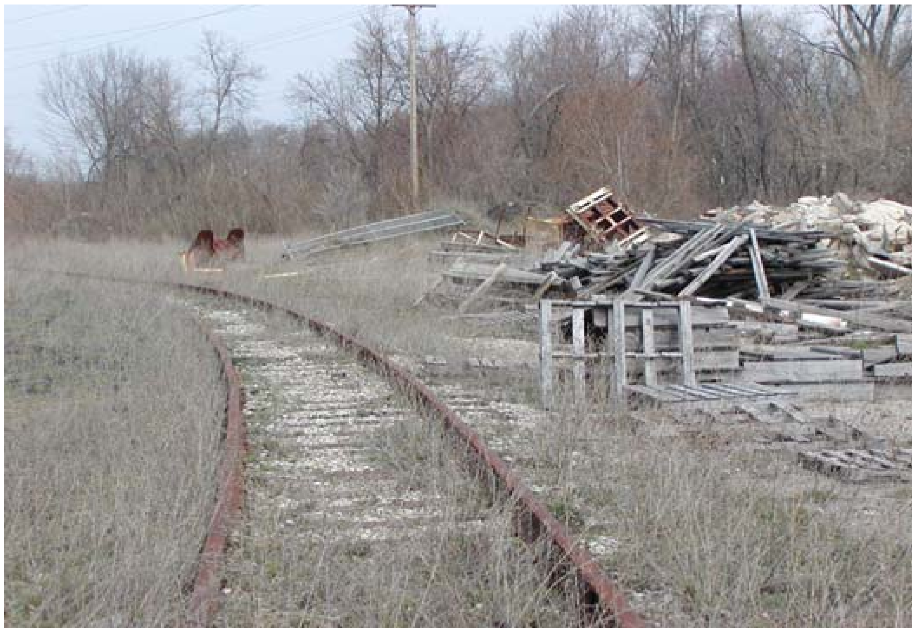
Existing Rail Line Extending Across Northern Portion of Plainwell Paper Mill Property
