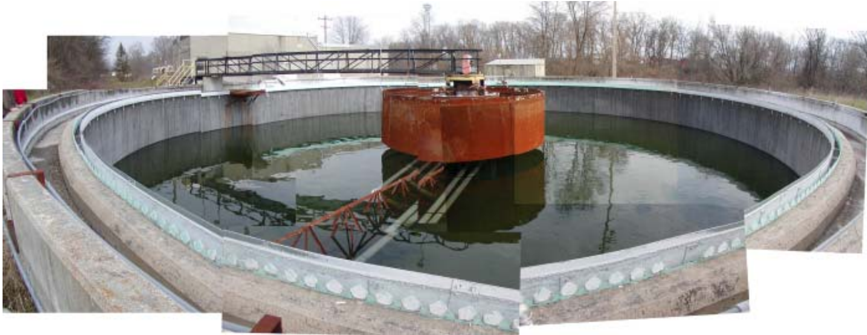
Existing Wastewater Lagoon
