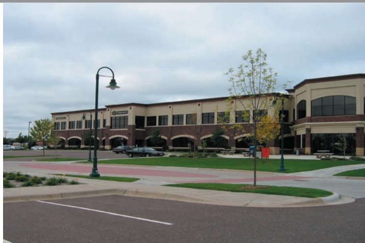
Office buildings at Brighton Corporate Park III
