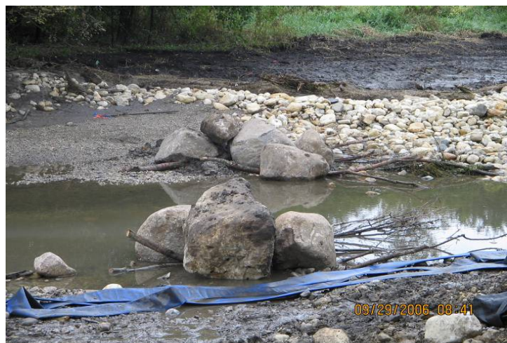
Restoration activities for the River OU included creating shoreline habitats along the streambanks. (Source: Wills Burke Kelsey Associates)
