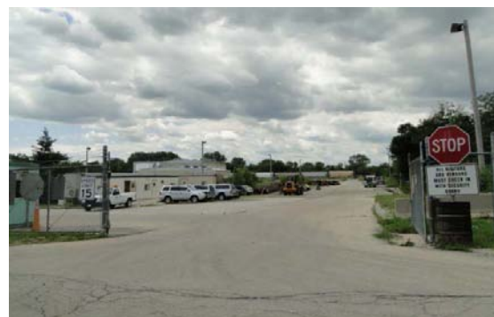
The REF serves as a transfer point for shipping radioactive wastes by rail to a licensed receiving facility in Utah. Note the rail cars in the background.
