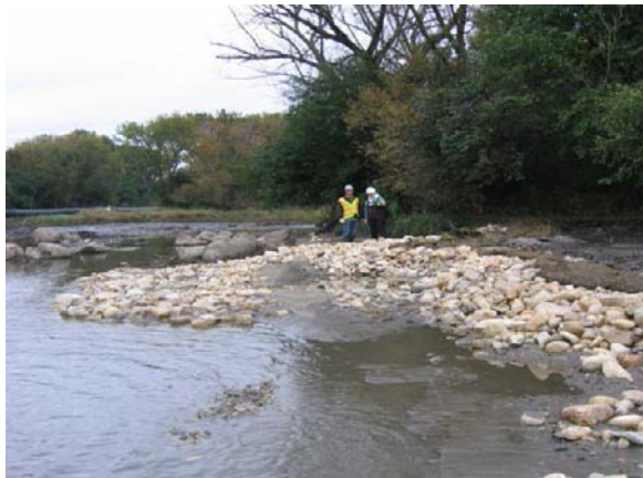
Ole Oldenburg and John Wills review the newly constructed floodplain which has been lowered in elevation with a crenulated cobble bank providing bank stability and habitat. (Source: Forest Preserve District)
