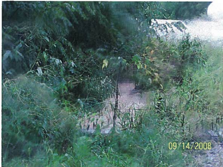
CULVERT NEXT TO THE HILLTOP ENTRANCE RAIN RUN OFF DRAINING INTO DITCH
